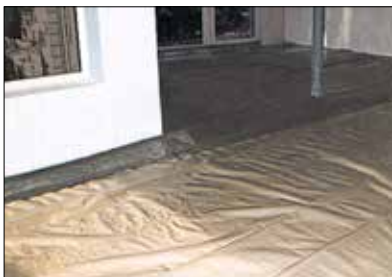
Installation of separating layer
