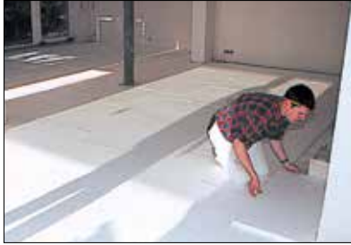
Installation of heat and sound insulation on a sufficiently load bearing and level substrate
