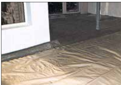
Installation of separating layer
